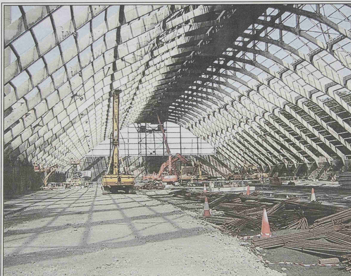
Construction is well underway; this photo shows the renovation of a Works' coal store into part of the terminal
