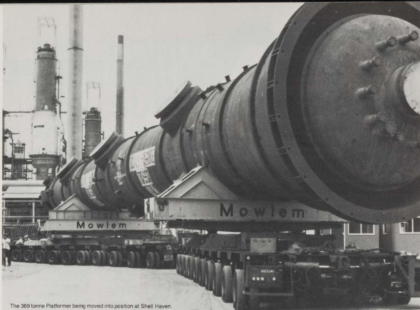
The 369 tonne Platformer being moved into position at Shell Haven.
