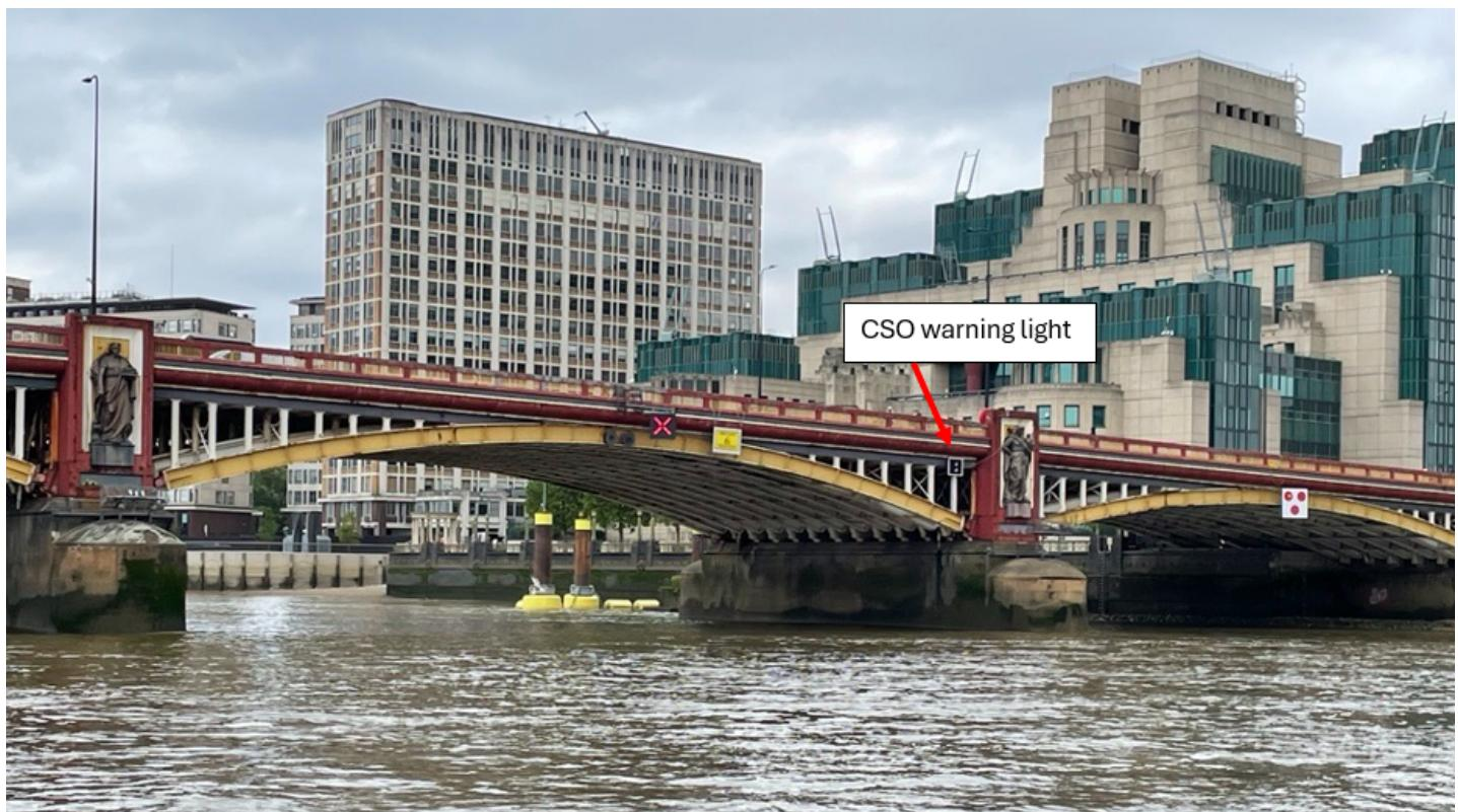
The lights will flash a yellow alternating 1 second pattern, visible day and night at a range of up to 200m, whenever the CSO is discharging or likely to discharge.
