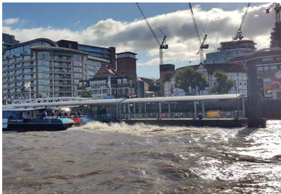
Bankside Pier - Unrestricted Berth
