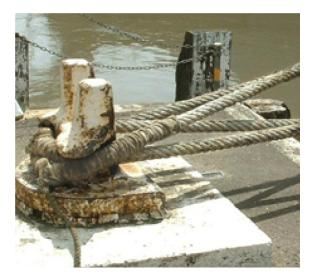
• All mooring lines on a bollard should be 'dipped' to facilitate prompt and easy release. Lines should only be "dipped" when slack, and when the weight of the line is held by another person or stopper. Where two Linesmen are so engaged, careful coordination between them is essential as the weight of the line is transferred to the bollard.
